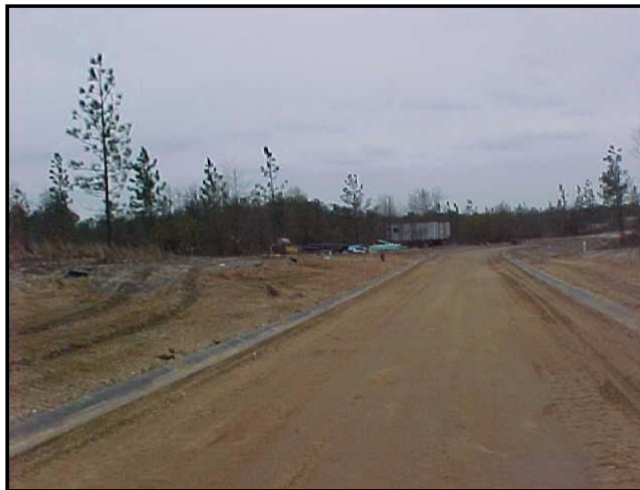
Looking at site
