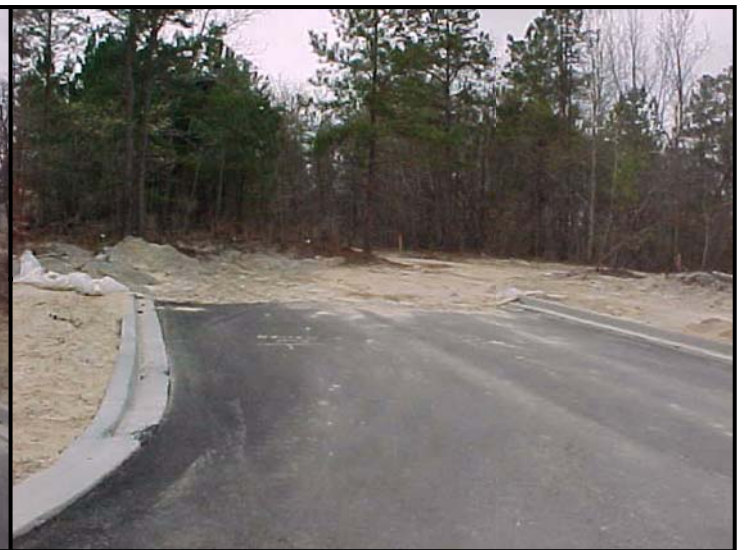
Looking at site
