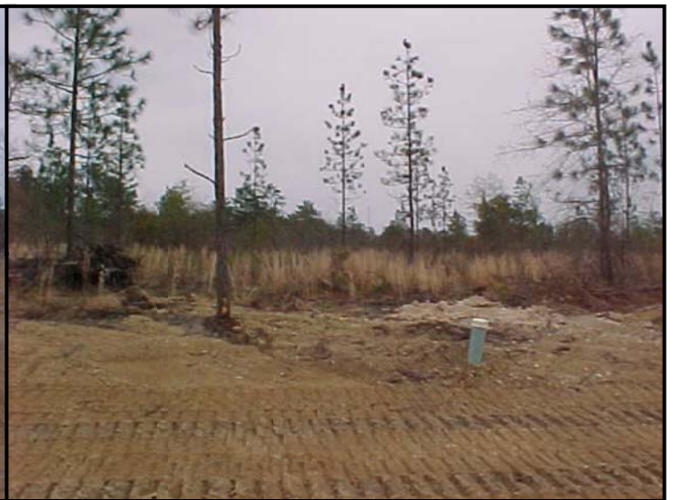
Looking at site
